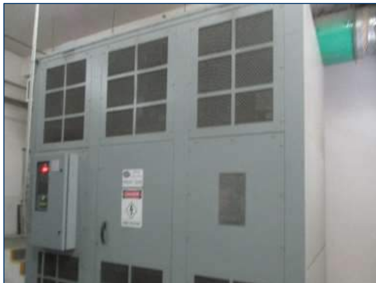
Electrical Switchgear Board
