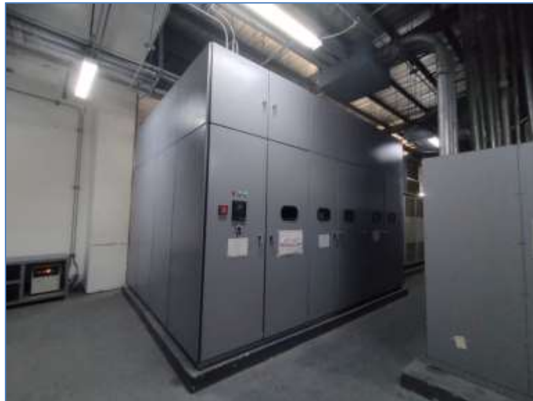
Medium Voltage Switchgear
