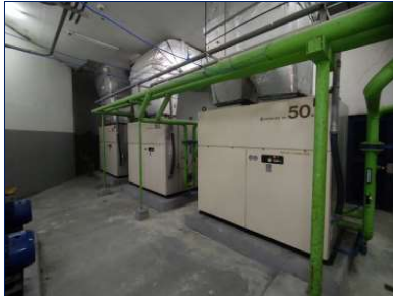
Package Air Conditioning Units
