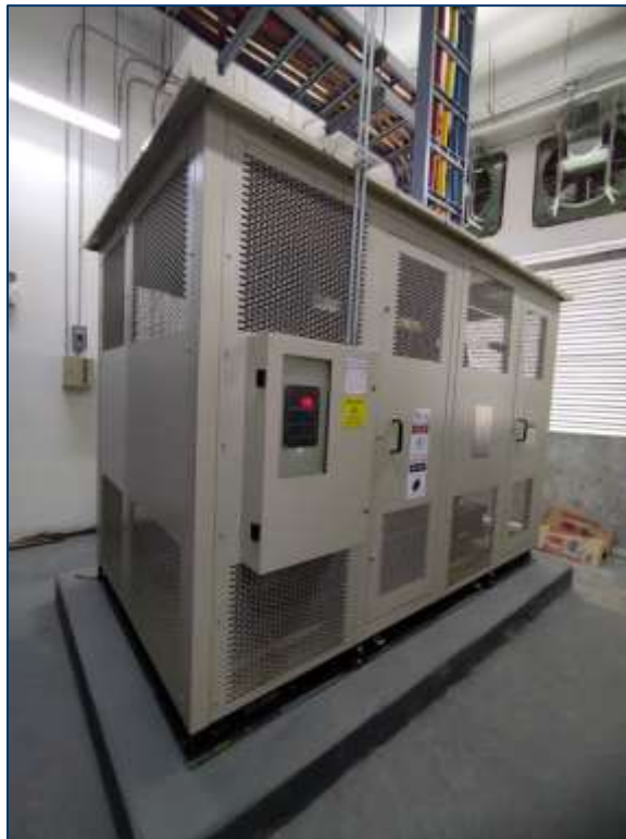
Distribution Transformer
