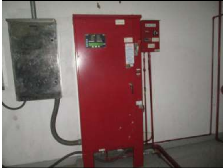
Fire Pump Controller and Jockey Pump Controller
