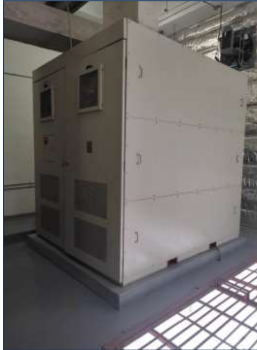
Power Distribution Transformer
