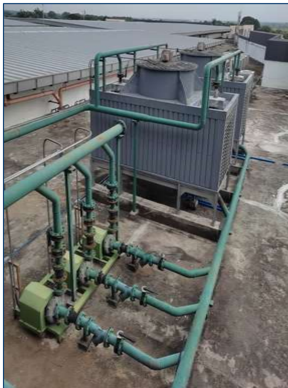
Cooling Tower Pumps and Cooling Tower
