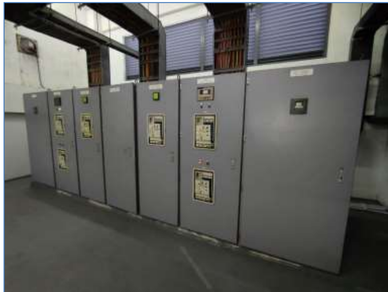
Low Voltage Switchgear Panel
