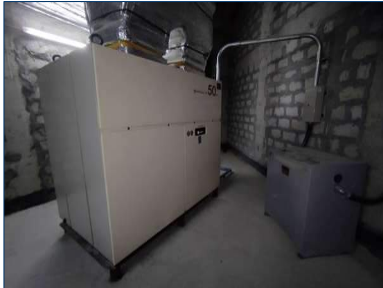
Package Air Conditioning Unit
