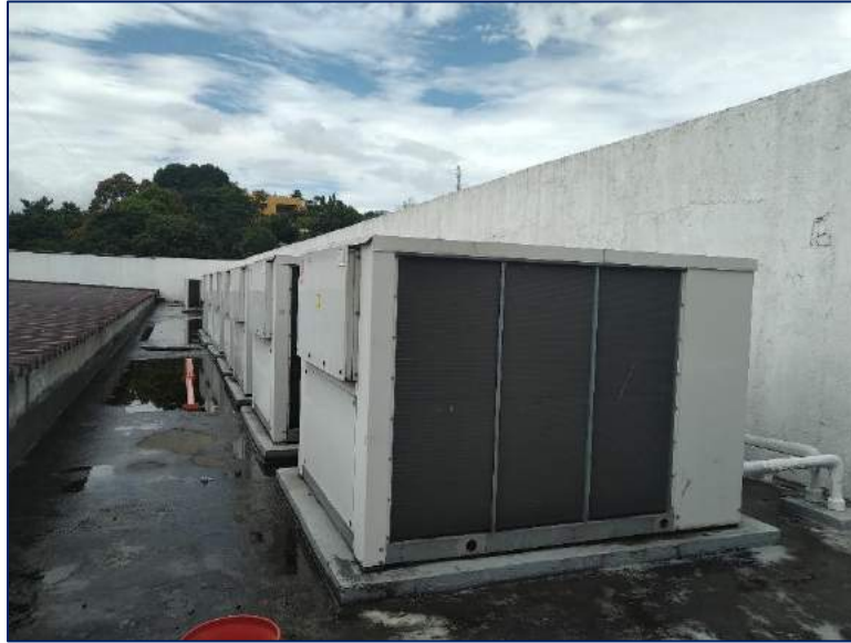
Air Cooled Condensing Unit
