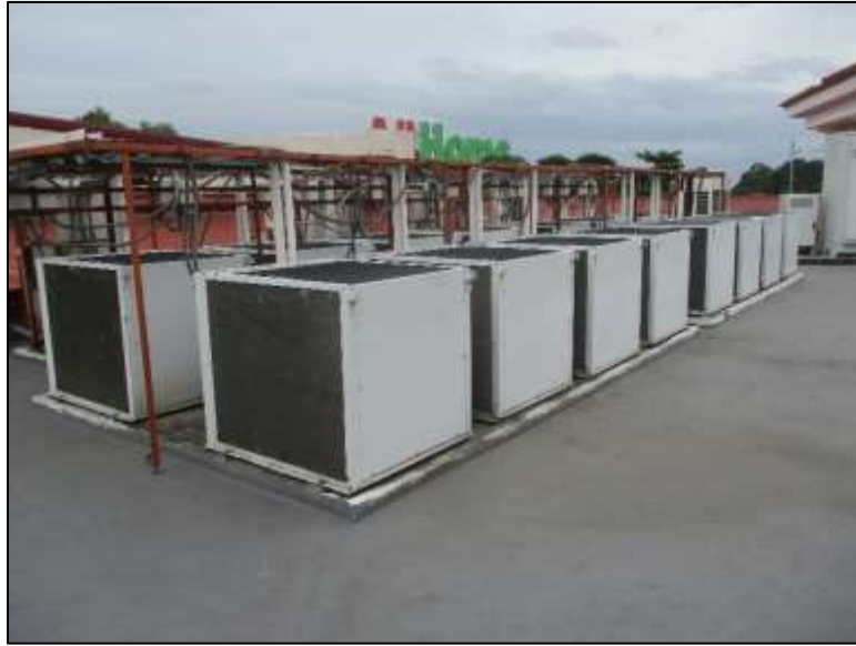
Air-Cooled Condensing Units
