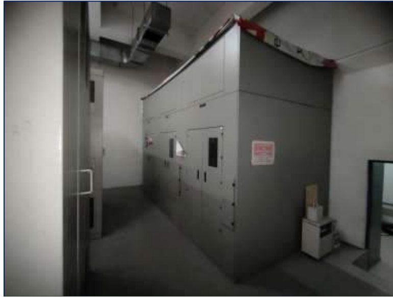
High Voltage Switchgear Panel
