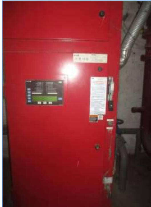
Fire Pump Controller
