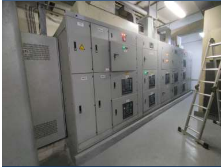
Low Voltage Switchgear Panel
