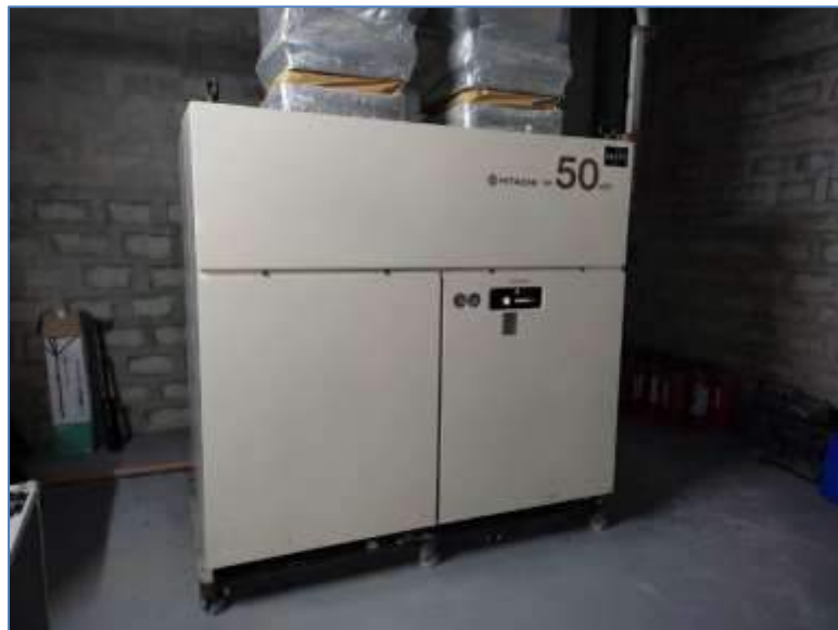
Package Air Conditioning Unit
