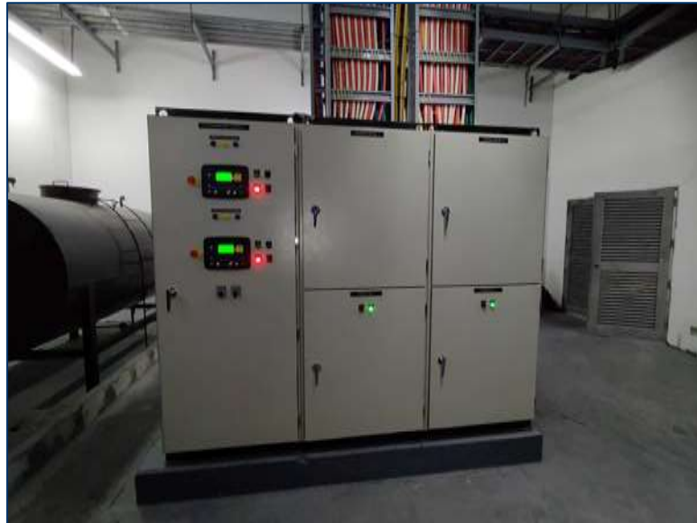
Generator Synchronizing Panel
