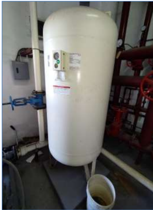
Hydropneumatic Tank
