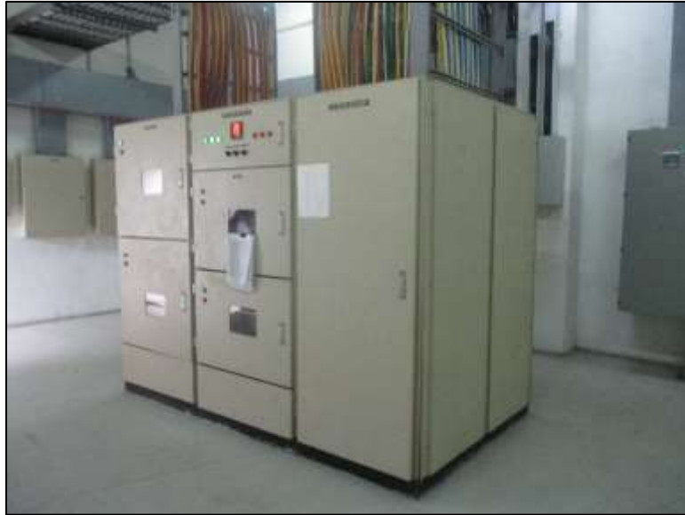
Automatic Transfer Switch Panel
