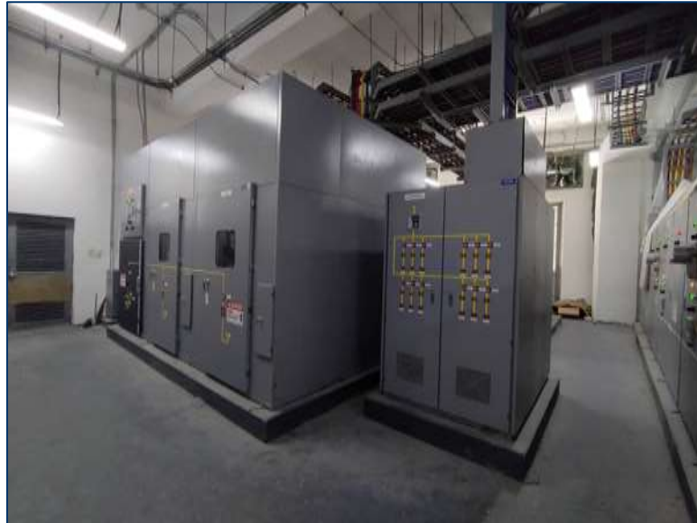
Medium Voltage Switchgear Panel and Capacitor Bank
